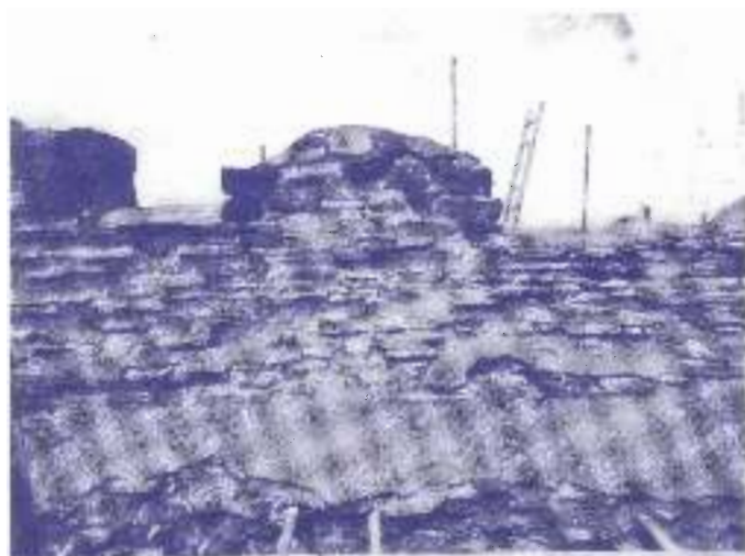
External side showing Merion no. 8 before repair showing the wall work before the core work was completed by the removal of the damaged masonry in the foreground.
