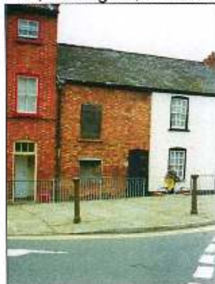
62 Castlegate before restoration
