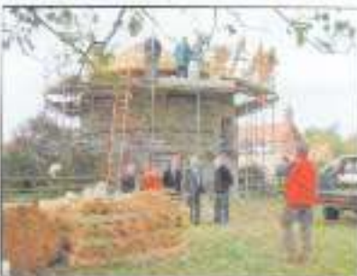
Above: A "watching installation" conducted by Mr Roger Scanlan
