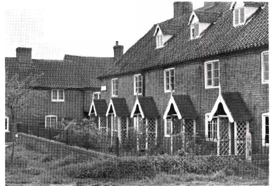
Sunnyside Cottages, Westthorpe, Southwell
