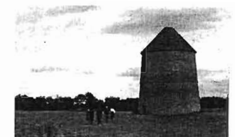
The Dovecote Tour in September 2012 enabled a small group of members to visit Flintham (picture above left) while restoration work on the ancient mud structure removed massive ancient ivy growth, and restored the walls and most of the nest holes using the traditional mix of mud, dung and straw. A canopy was later erected to protect what remains from the elements. After a visit to Thoroton, the group moved on to the massive dovecote at Sibthorpe, (picture above right) now owned by Nottinghamshire County Council.
